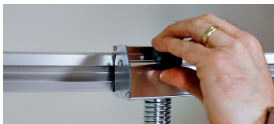
6 Fasten the profiles with the screw.
